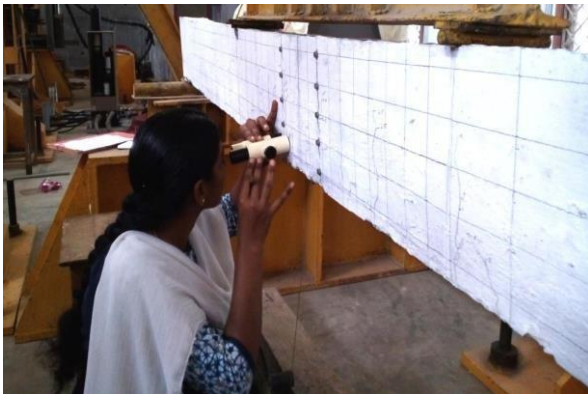
Fig. 4.50 Measuring Crack Width using a Crack Detector Microscope
