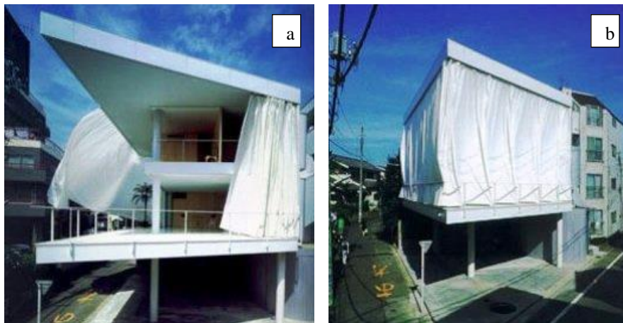
Figure 22. Curtain Wall House, 1995, Tokyo, Shigeru Ban, a: without curtains; b: drawn curtains.
