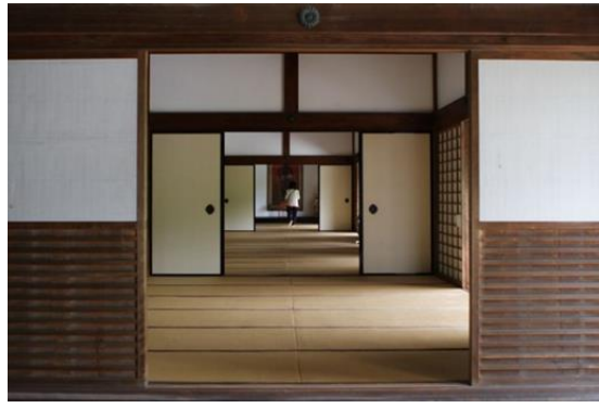
Figure16. shoji, removable partition between rooms.
