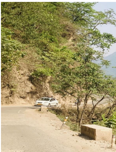
(Fig 1) Landslide prone area
