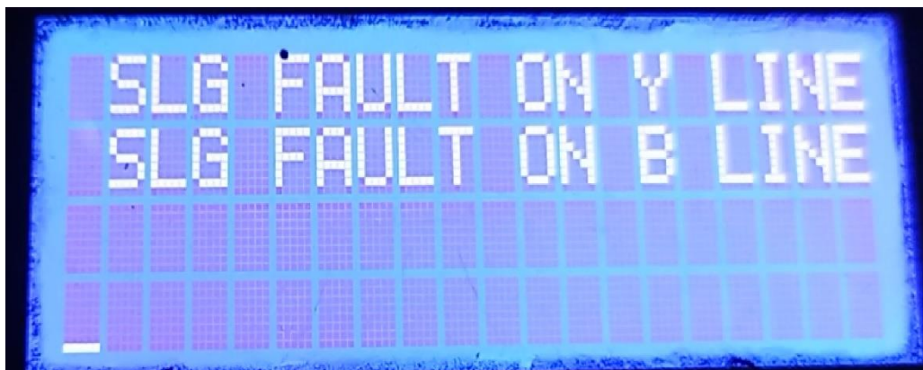
Figure 9.LCD display showing fault details of LLG fault
