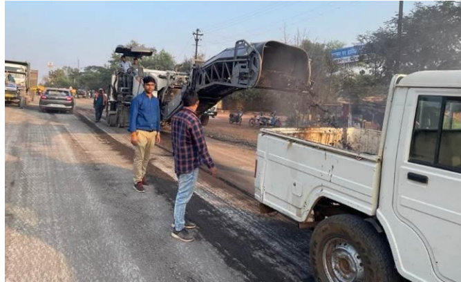
Figure 2.1: Cold Removal Process (control-Depth) in NH-53 Ch 345+200 (Rajnadgaon, Chattisgarh)
