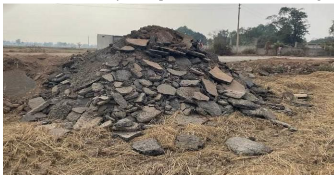
Fig. 2.3 Site dumped RAP material (full-depth demolition) at Chandrapur-Dabhra State Highway
