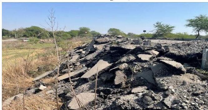
Fig. 2.2: Site dumped RAP material (full-depth demolition) at sarangarh - Baramkela S.H.
